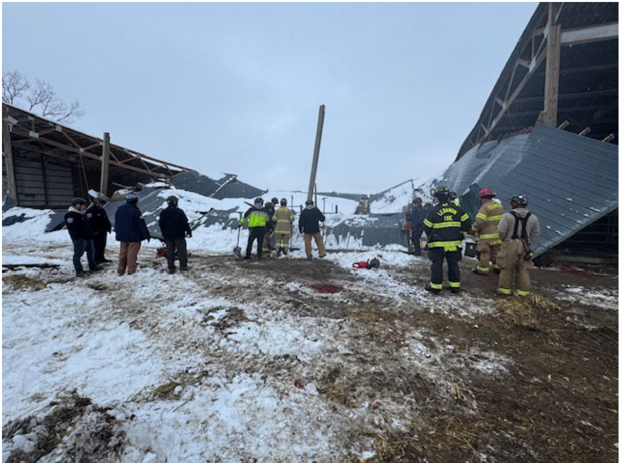
( Barn Collapse Waynesville )
